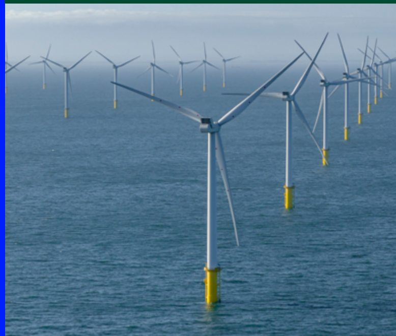
Image courtesy of Greencoat UK Wind
